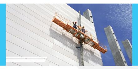
Horizontal Wall Elements are reinforced wall elements that can be used both in interior and exterior wall frame gaps formed by reinforced concrete, steel, wooden or prefabricated structure framework. These elements can be mounted to the interior and exterior surfaces of the colomns as well as between the columns.
