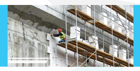
AAC Thermal Insulation Plate having a thermal conductivity value of 0,05 W/mK, is a mineral-based, massive and non-combustible thermal insulation material.
