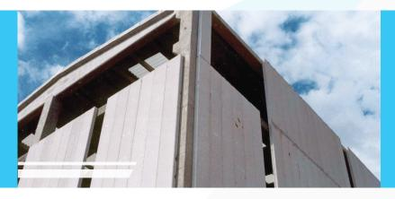
Vertical Wall Elements can be used as interior and exterior walls in structural frame gaps formed by the structural framework, or can be used as a partition wall independently from the framework.
