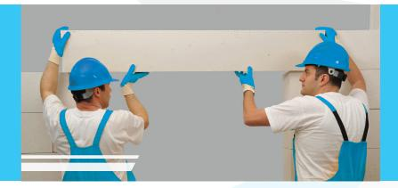
Lintel sizes are determined according to the size of wall blocks, therefore they don't have any fitting problems. During assembly, AAC Lintels must be placed upon adhesive mortar. Utmost attention shoud also be paid to keep the overlapping allowance not less than the assigned measures
