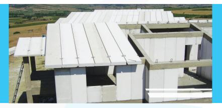
AAC load-bearing vertical wall elements can be used as both interior and exterior walls in masonry constructions. AAC floor deck elements are used as slab, whereas in roofs, AAC roof elements are used.
