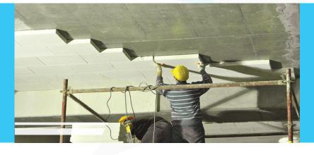
AAC Thermal Insulation plates are used for hea insulation of exterior facade, ceiling of basements and carparks as well as for heat insulation of terraces and roofs.
